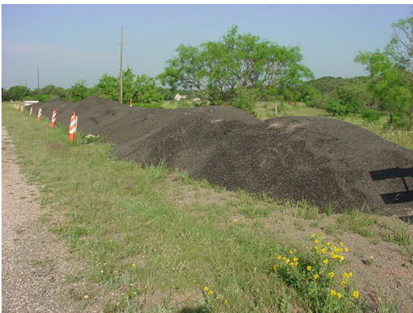
Figure 6-1. Properly Placed Aggregate Stockpiles.
