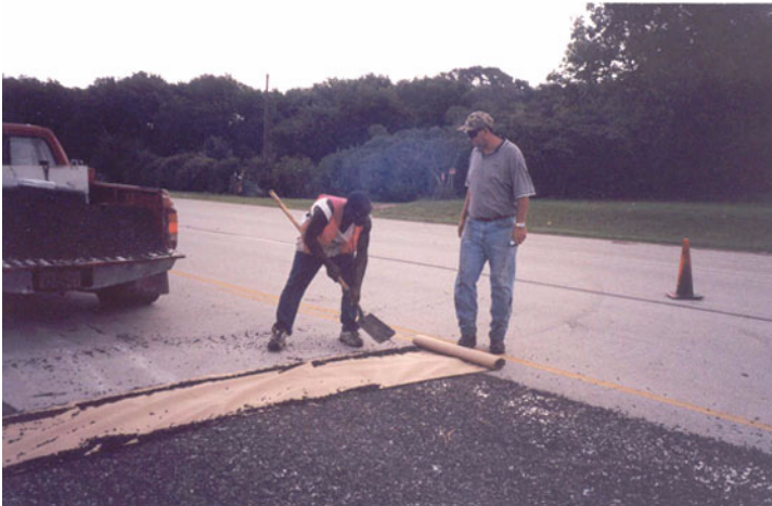
Figure 8-3. Placing a Paper Joint at Beginning of Shot.
