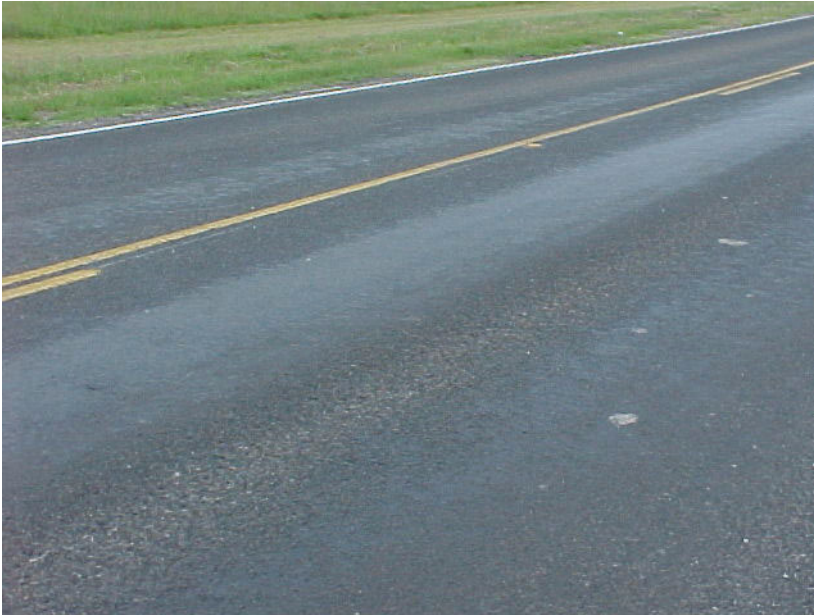
Figure 1-2. A Seal Coat Pavement Surface Exhibiting Flushing in the Wheelpaths.
