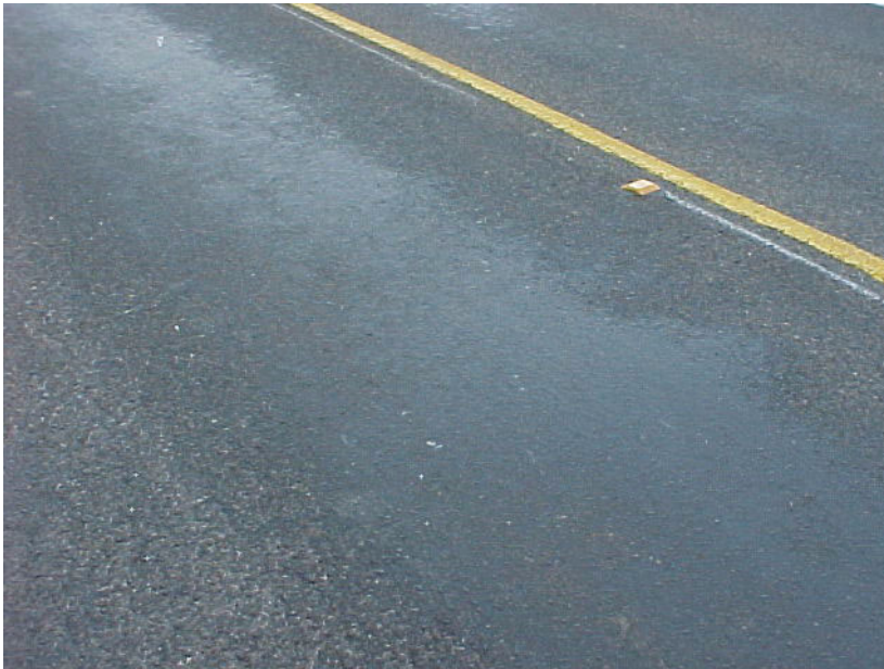
Figure 1-1. Seal coat pavement surface exhibiting aggregate loss.
