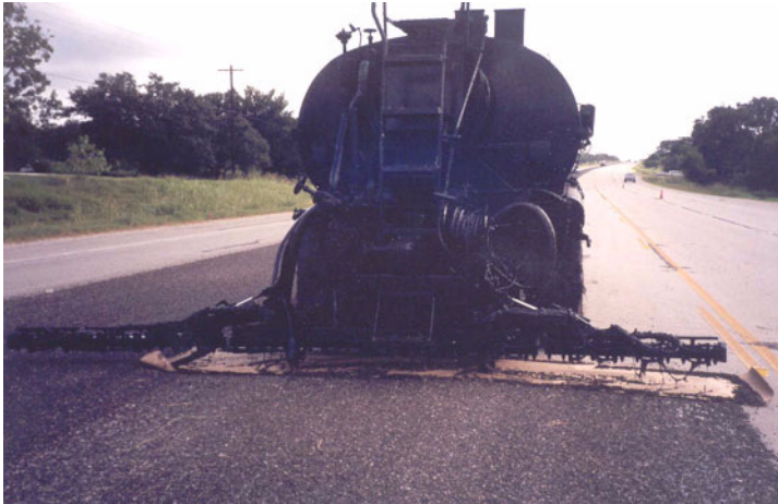
Figure 8-6. Correct Starting Position over Paper Joint.
