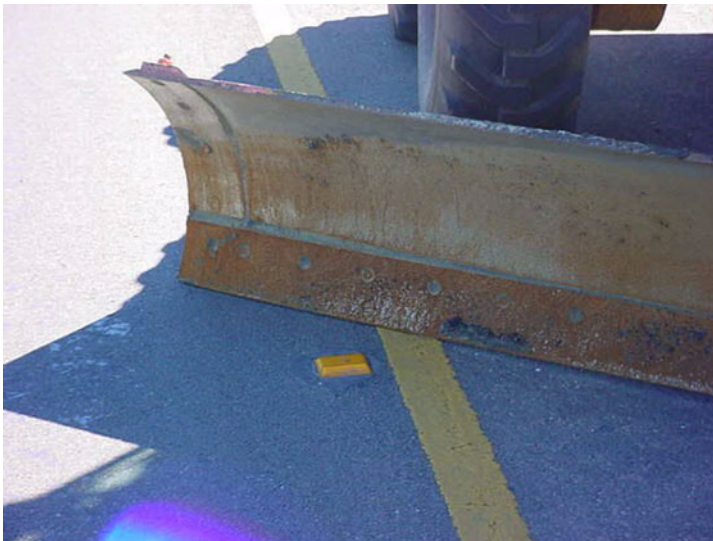
Figure 8-2. Removal of Raised Pavement Markers.
