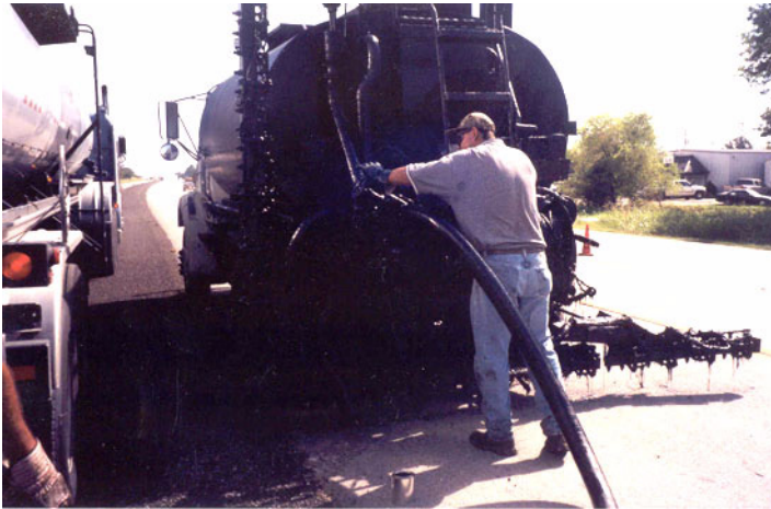
Figure 8-5. Transferring Asphalt from Transporter to Distributor.
